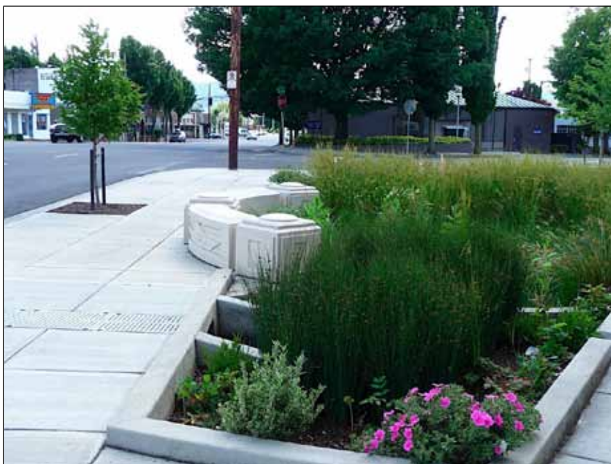
Stormwater planter in the public right-of-way, Portland, Oregon.
