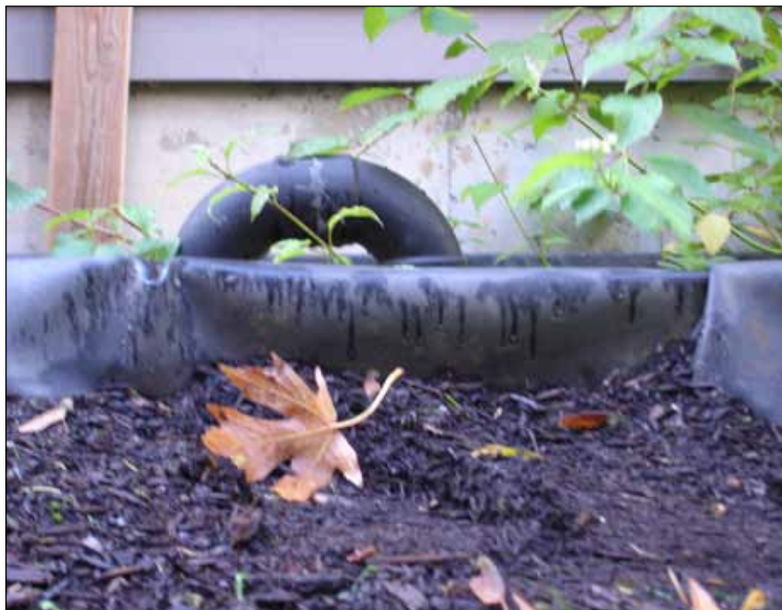
Improperly installed U-shaped overflow.
