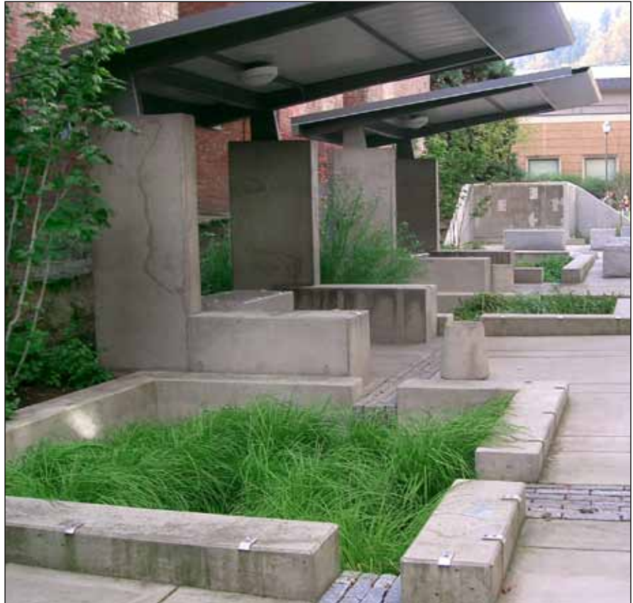
Stormwater planter at Epler Hall on the Portland State University campus.
