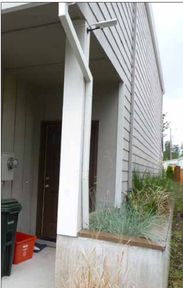
Filtration planter built into a private residence, Mignonette Estates, Gresham, Oregon.
